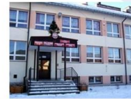
Community Kindergarten in Jurków
